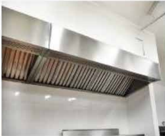
SS EXH. HOOD W-FRESH AIR (2)
